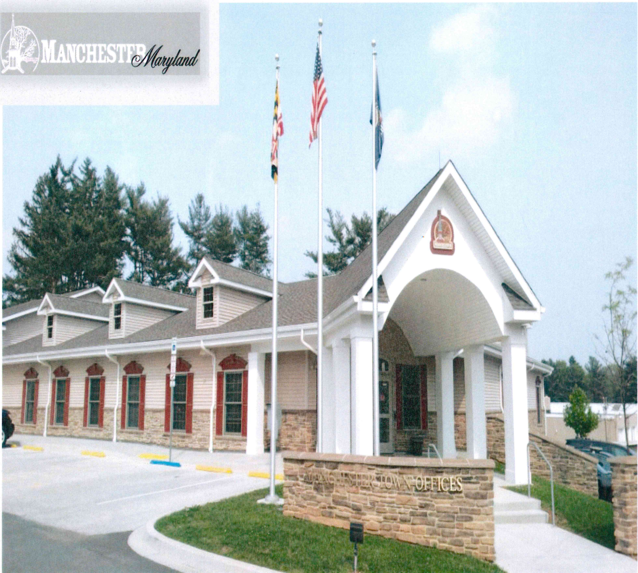
Manchester Town Offices and Police Station
